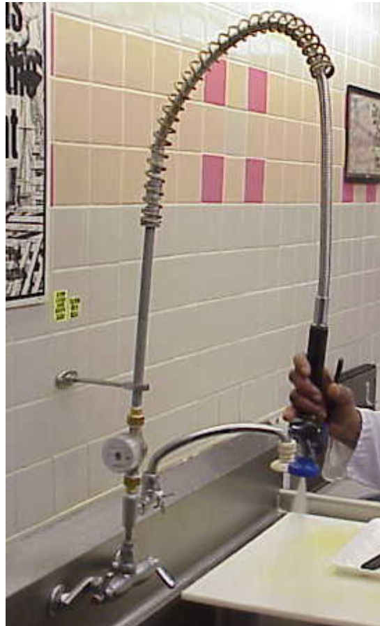
Figure 3: Metering setup for determining hours of use
