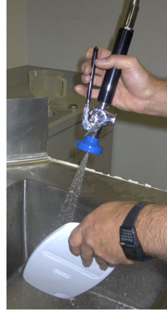
Figure 1: Low-flow pre-rinse spray valve in use
